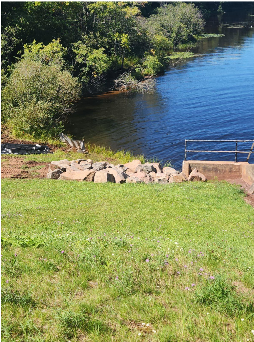
Figure 4. West Wingwall Repair
